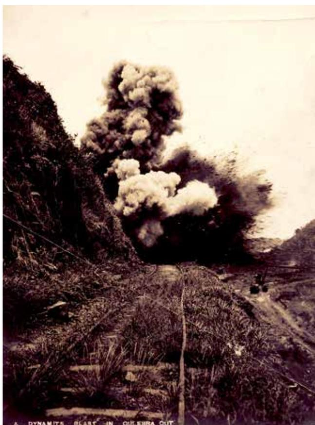
Dynamite blast during excavation of Panama Canal, ca 1904–1914
