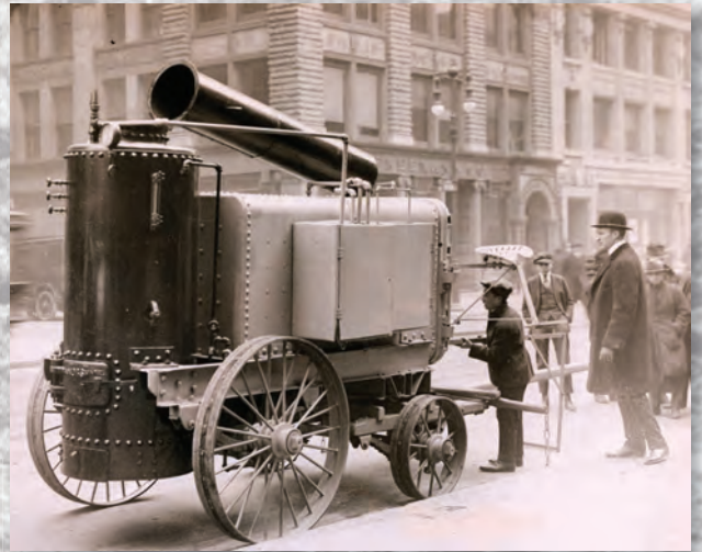
Lice that spread epidemic typhus were a serious concern on the front. This 8,000 pound steam sterilizer could kill those "cooties," as the soldiers called them, on the gear of forty men at a time.
