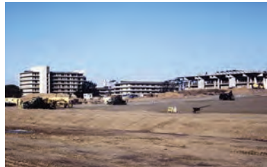
UCSD Revelle College campus under construction, 1964 Charles H. Graves Photographs and Films, UCSD
