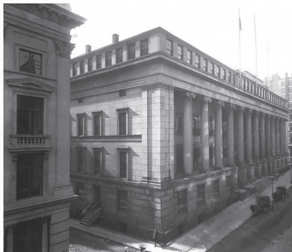
Weil’s father worked as a customs broker at the Merchant’s Exchange Building (now the National City Bank Building) at 55 Wall Street. Photo ca. 1899–1919. New York Historical Society
