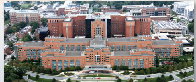
Aerial view of the Clinical Center, NIH, 2014 NIH
