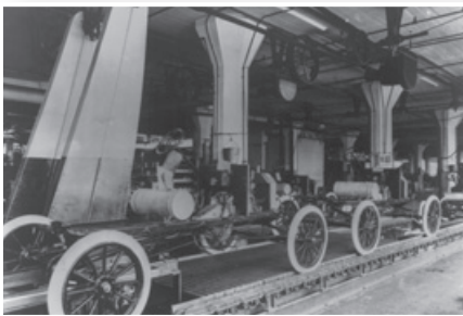
Early moving assembly line at Ford (ca.1913) Library of Congress, Prints & Photographs Division
